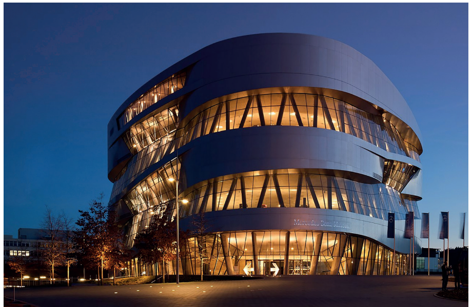
The 47m high façade of the Mercedes-Benz Museum in Stuttgart is coated in Monopol paint
